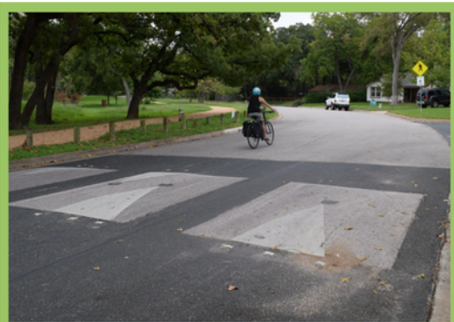
Asphalt Speed Cushion
