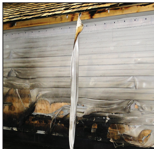
This vinyl gutter melted from heat, exposing the wood and roof edge to embers and direct flame. Photo by Institute for Business and Safety Research Center.
