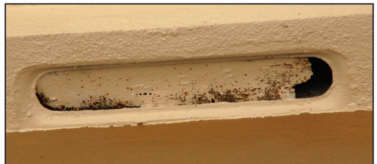
Vents can clog. This vent was painted over, reducing its effectiveness in providing ventilation. Photo by Institute for Business and Safety Research Center.
